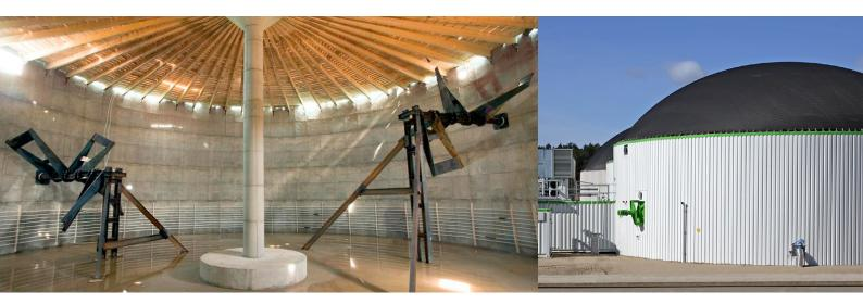
The REMEX<sup>®</sup> agitator operates continuously, evenly mixing substrates in the biogas plant's digester or post-digester while protecting the process biology.
